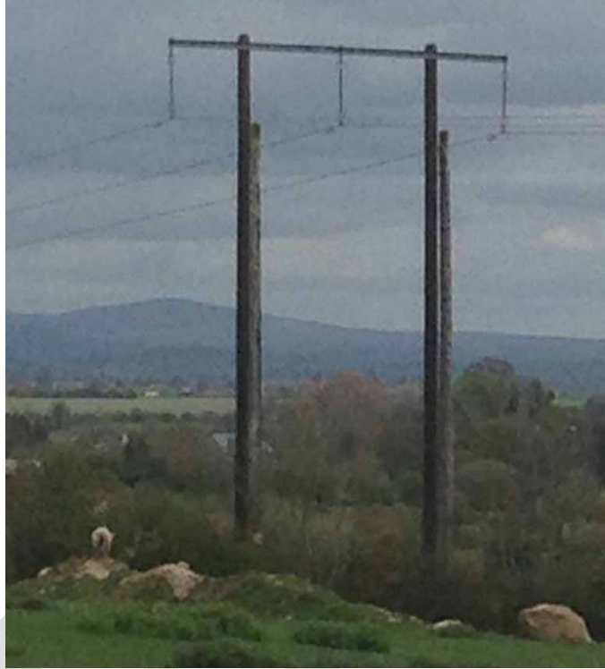
Figure 2-1: Example of existing 110 kV poleset being replaced with new and taller poleset (old poles still to be removed)
