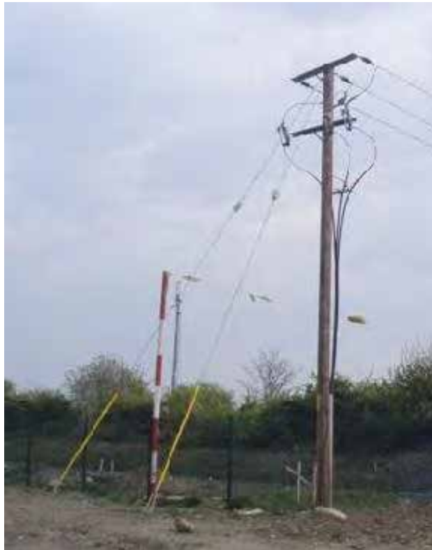
Figure 3-1: A typical MV line/cable interface pole
